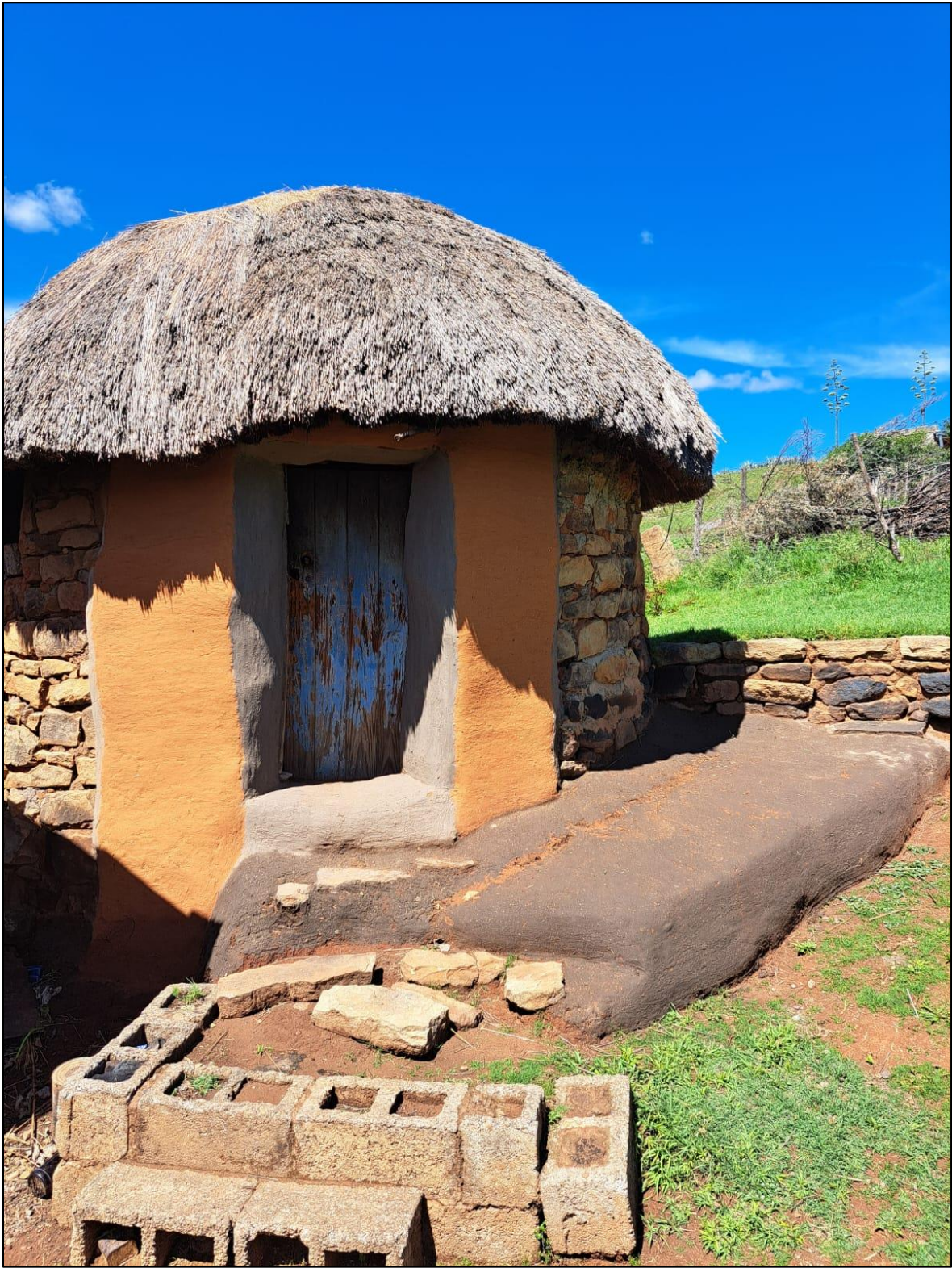
D – Sample of a Basotho Traditional House – a hut (mokhoro)
