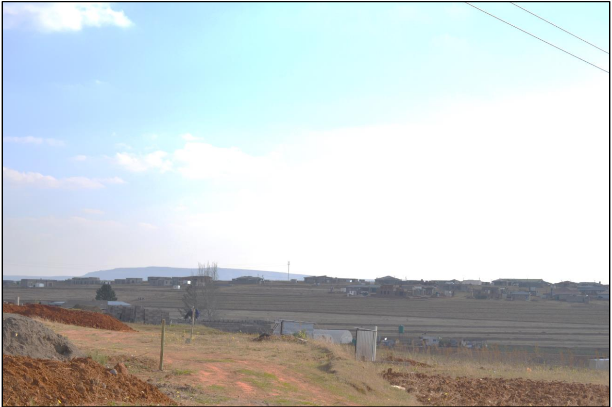
Figure 5.26 SBIH development encroaching on agricultural land at Ha Motloheloa, Mohlakeng Community Council
