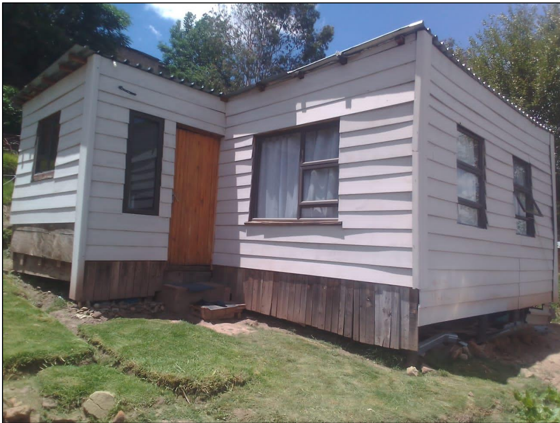
Figure 5.21 A start-up temporary SBIH at Maseru Municipal Area, Maseru AD
