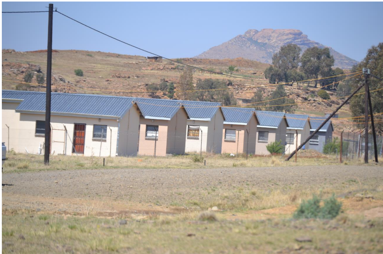
Figure 5.19 Affordable housing scheme by LHLDC, Mafeteng Urban Council, Mafeteng AD
