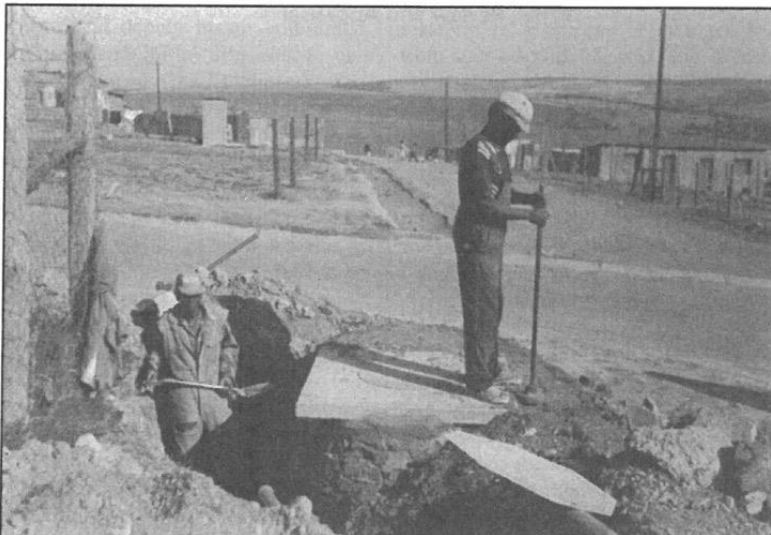
Figure 5.3 Construction of sewerage lines in Mlungisi (Nussbaum, 1997: 73)
