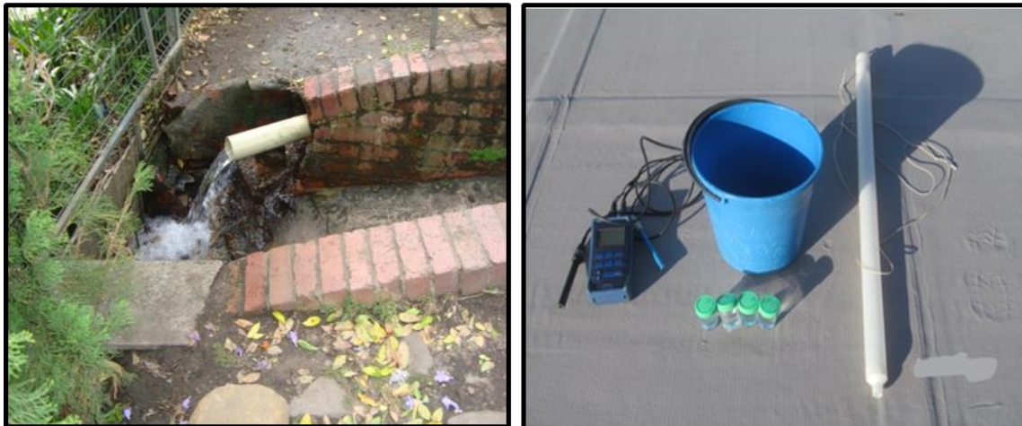
Figure 14. Newlands spring water piped from the source, using a PVC pipe.
