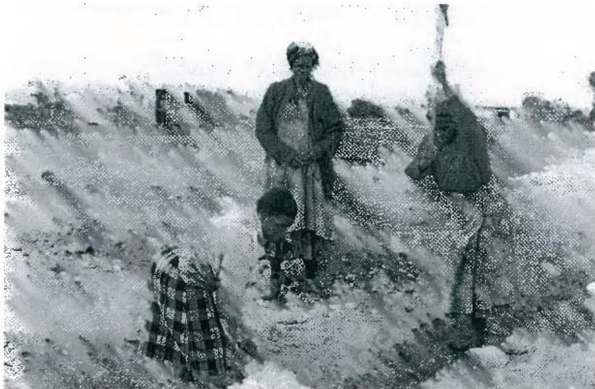
Women digging the first foundation
