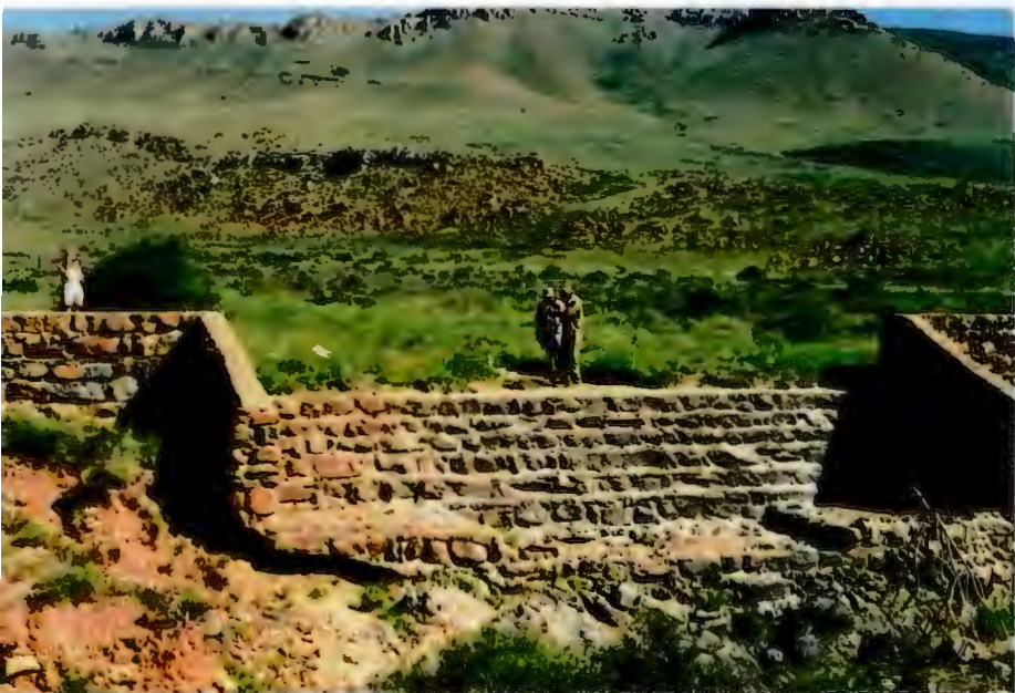
Plate 10.2 Uppermost weir on the Klein Seekoei River. Note the state of vegetation rehabilitation on the valley floor.
