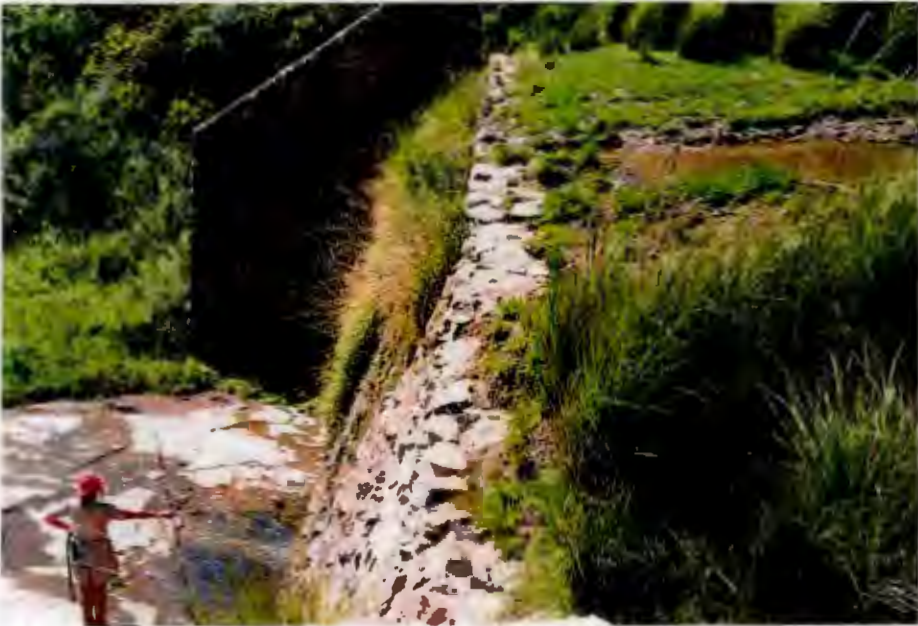
Plate 6.5 Stone and concrete weir on the upper Klein Seekoei River, circa 1948. The weir, one of four in this segment of the catchment, was constructed as an anti-erosion mechanism.
