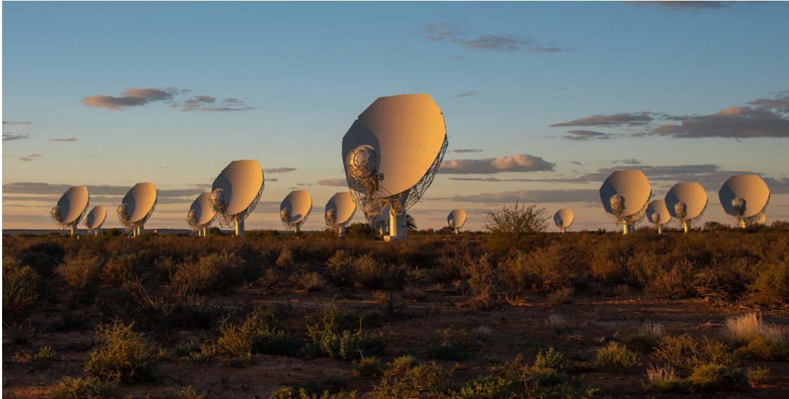
Figure 1.4: The MeerKAT radio telescope during inauguration in July 2018. Only part of the array is shown in the image, with the Gregorian offset configuration design of the antennas in display. Image sourced from: SARAO MeerKAT Array .
