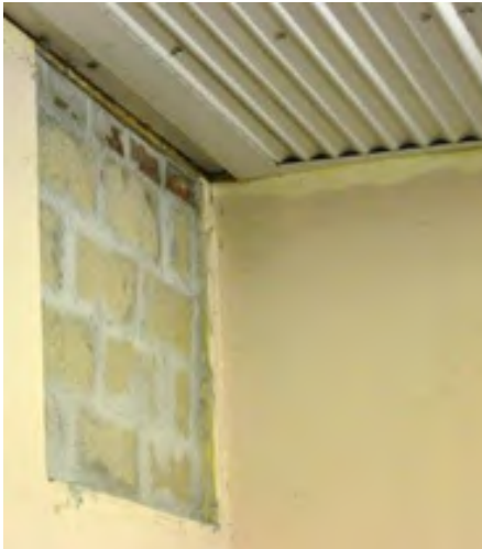
Figure 52: Bonteheuwel Secondary School: Photograph to show kitchen window which has been bricked-up due to theft problems
