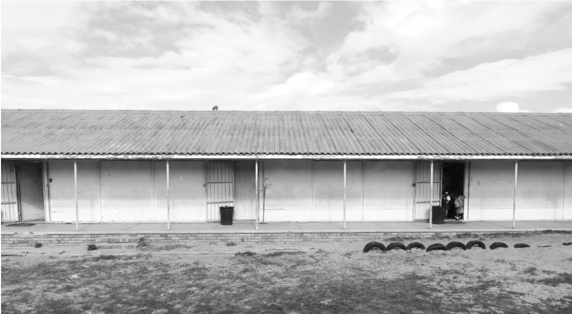
Figure 2: "All the school reforms on earth are worthless if kids have to come to school in buildings that destroy their spirits." (Lackney, 1999) This photograph, showing the impoverished experiential quality of a school in Grassy Park, seems to illustrate Lackney's statement
