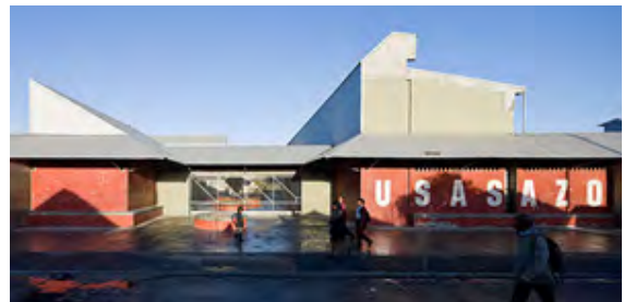
Figure 31 [top]: Usasazo Secondary: Photograph to show street view of school (still frame from documentary by Southwood, 2010)
