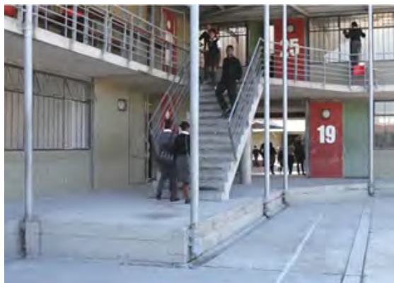
Figure 27: Usasazo Secondary: Photograph to show stairs and walkways as places for social interaction (still frame from documentray by Southwood, 2010)
