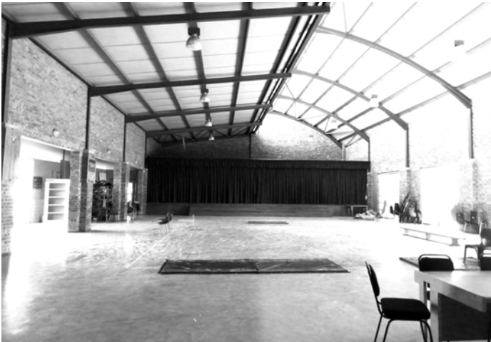
Figure 30: Wesbank No1 Primary: Photograph to show multi-purpose hall
