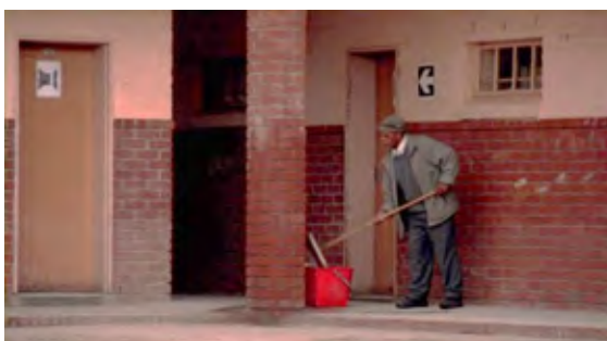
Figure 60 [below]: Masipumelele Secondary School: Still-frames from ‘Schools that Work’ documentary to show facebrick walls being scrubbed down by the caretaker (Jansen & Blank, 2014)
