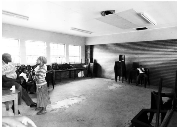
inadequate forum space
