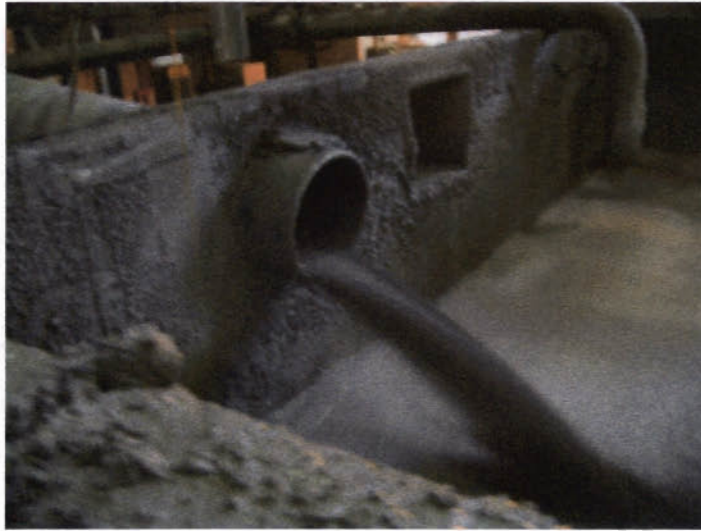
Figure G-4 A stream with possible segregation across a pipe
