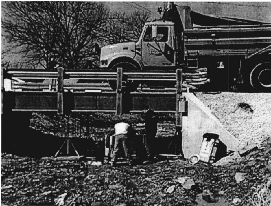
Figure 5. St. James Bridge (Nystrom et al., 2003)
