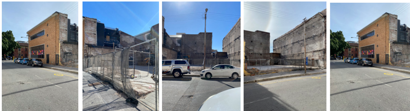
Figure 35: Site current condition
