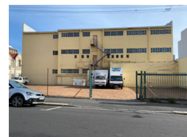
Figure 36: Side view from Harrington Street
