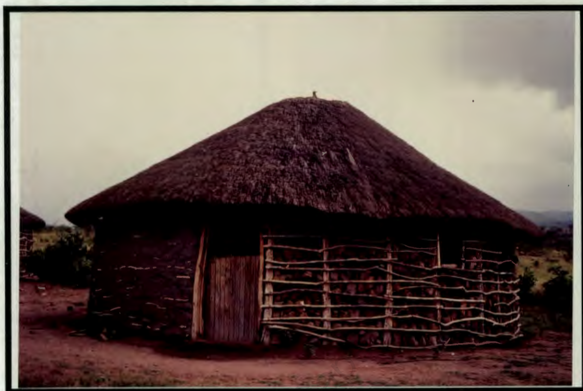
Plate 4.6 Dwelling under Construction
