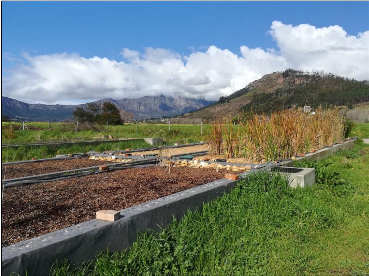
Figure 4.6: Peach pip and small stone biofilters at the Water Hub
