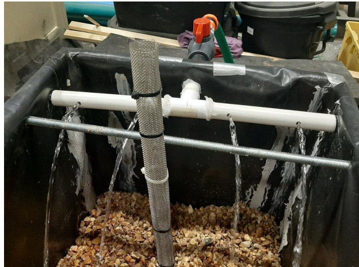
Figure 5.6: Pilot biofilter inlet (photographed during construction)
