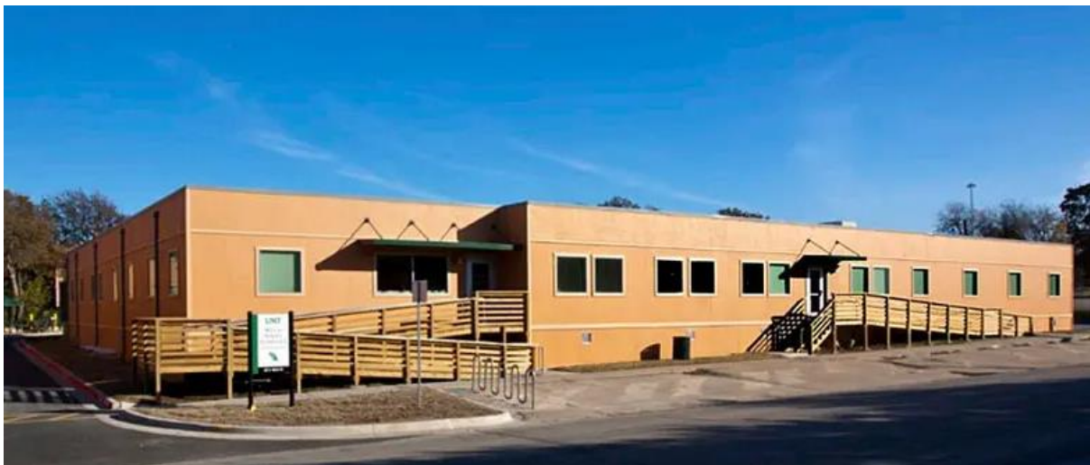
Figure 3: The construction of a 1300m 2 office building (Ramtech Building Systems, 2013)
