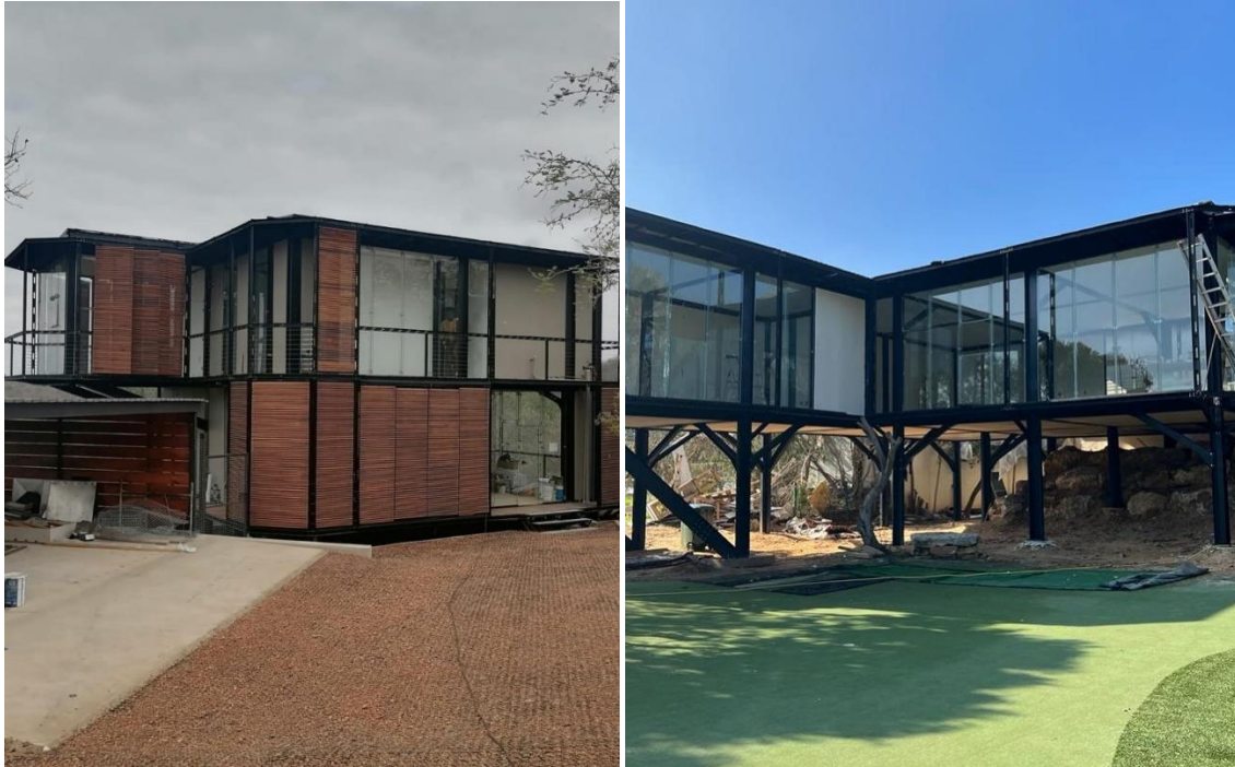
Figure 2: Residential home designed and constructed in South Africa (HouseZero, 2022)
