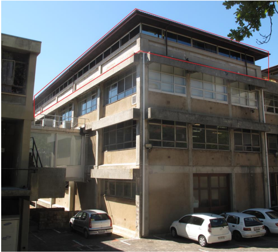
Figure 1-1: North-west corner of Menzies; the ERC exterior, on the top floor, is highlighted within the red lines
