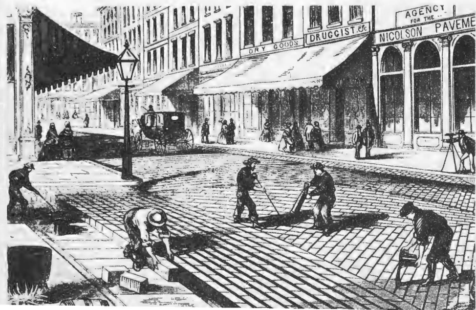
Fig. 41 Laying Nicholson Pavement 1859
