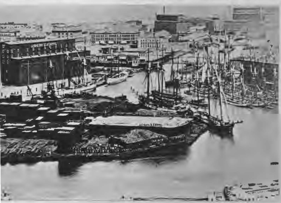
Fig. 61 Rebuilt Chicago River Area 1875
