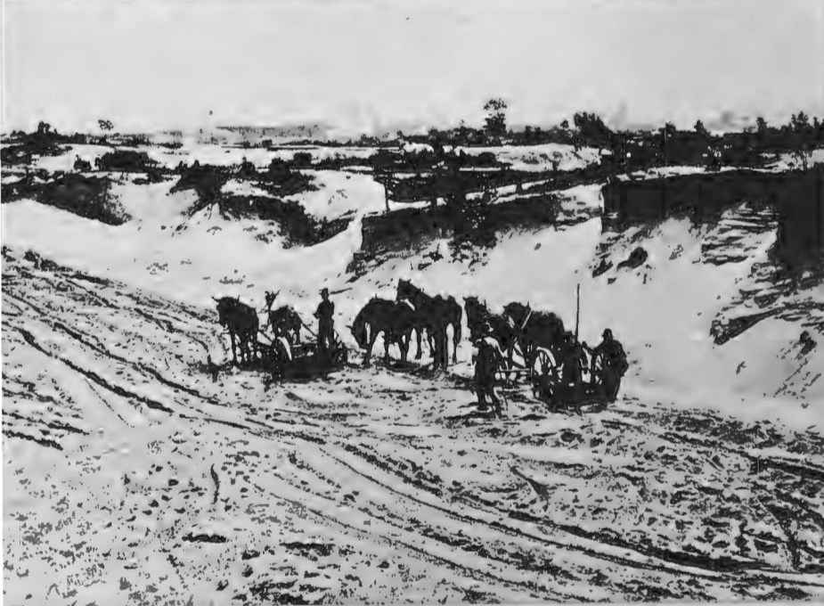
Fig. 115 Site Clearing for Steel Works, Gary 1906
