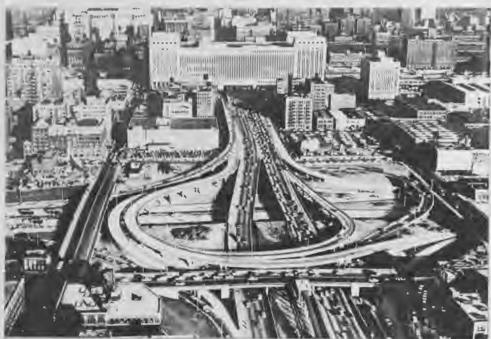
Fig. 145 Chicago Circle Traffic Interchange 1961
