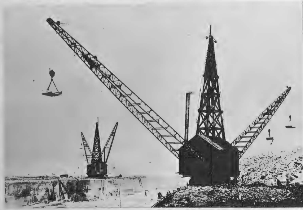
Fig. 116 Construction, Sanitary and Ship Canal 1899
