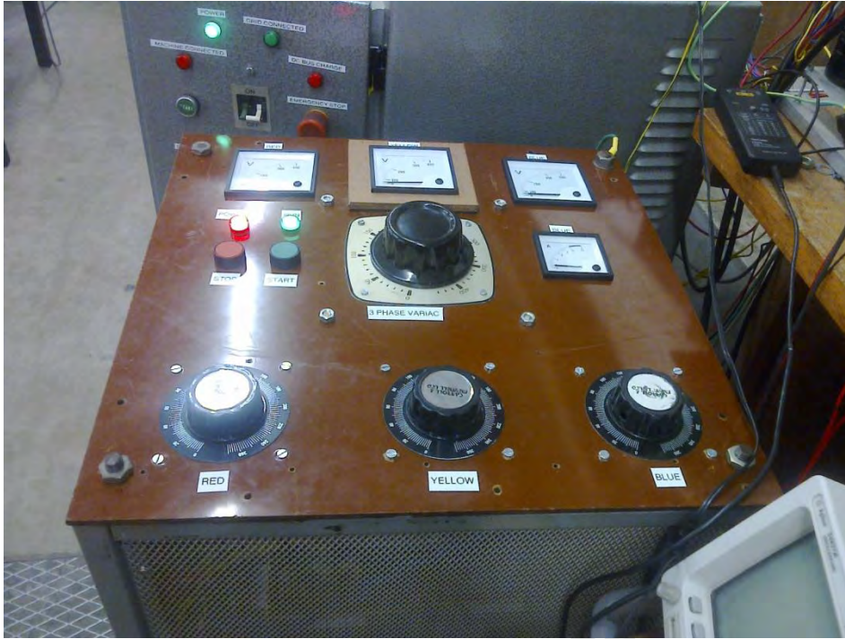
Figure 5.45: Three phase variac used to implement voltage unbalance
