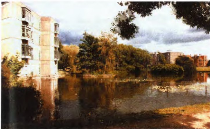
6.9 York University View across lake of Langwith College showing CLASP system of construction [Muthesius, 2000]
