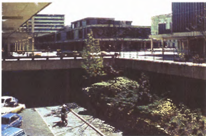
6.28 Bath University View of Parade with service road below
