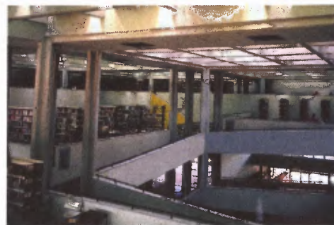
6.97 University of Zambia Interior view showing ramped access to floors at 800mm. intervals
