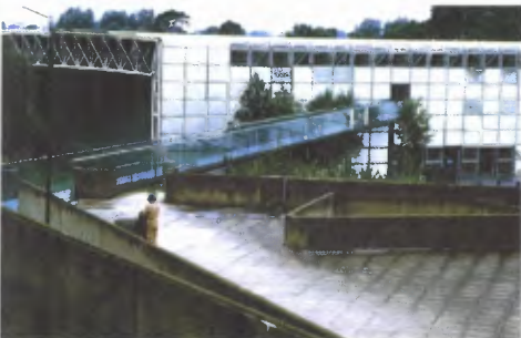
6.15 University of East Anglia Western end of walkway now terminated by 'high tech' building housing Sainsbury Colletion
