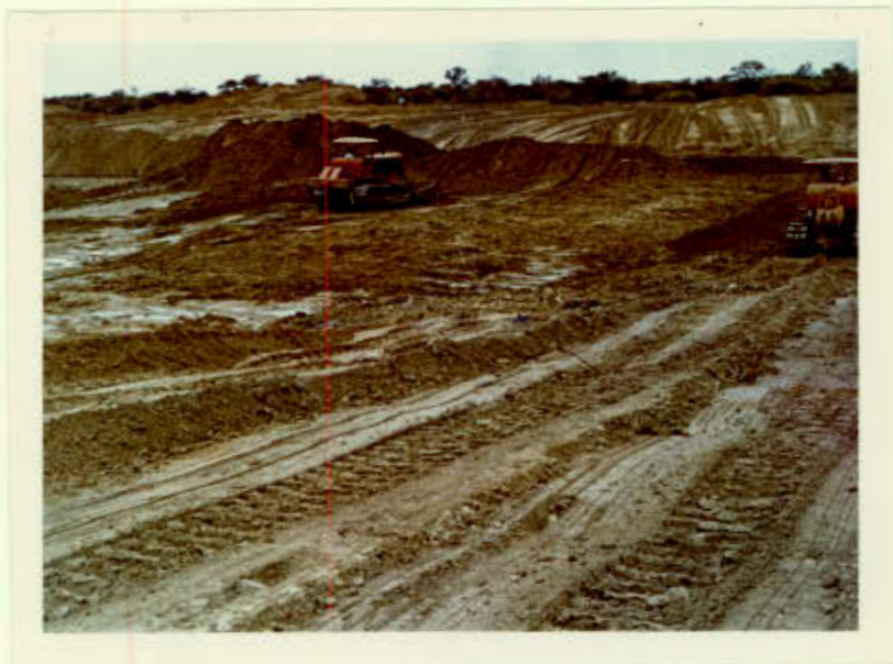
Photo 8 : Quartzose lateritic gravel near Suk-ses being stock-piled for use in the basecourse. Note standing water due to poor drainage conditions.
