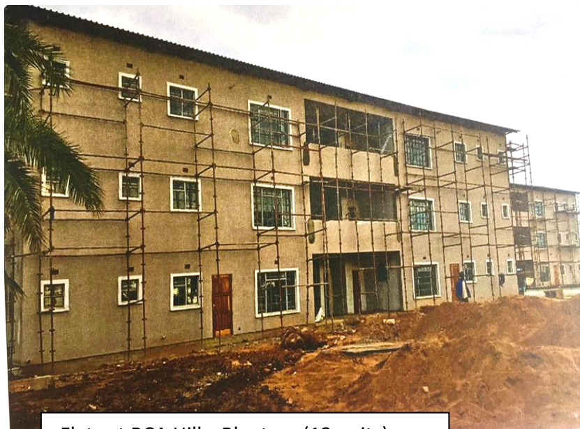
Flats at BCA Hills, Blantyre (12 units)
