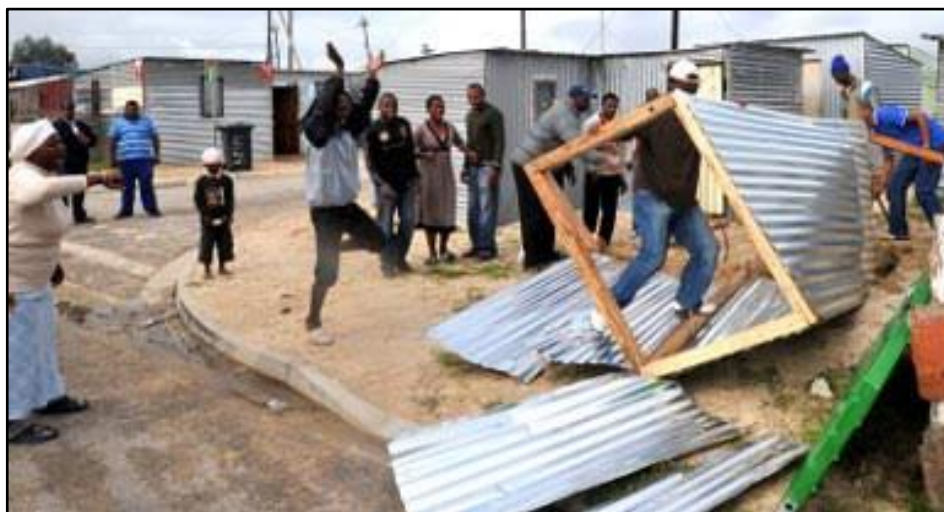
Figure 3: Dismantling the zinc toilet covers (Honwana, 2010)
