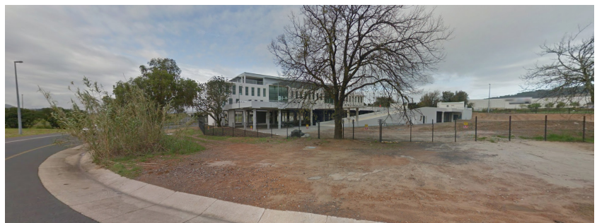
21: STREET VIEW OF CECILIA STREET OFFICE PRECINCT
