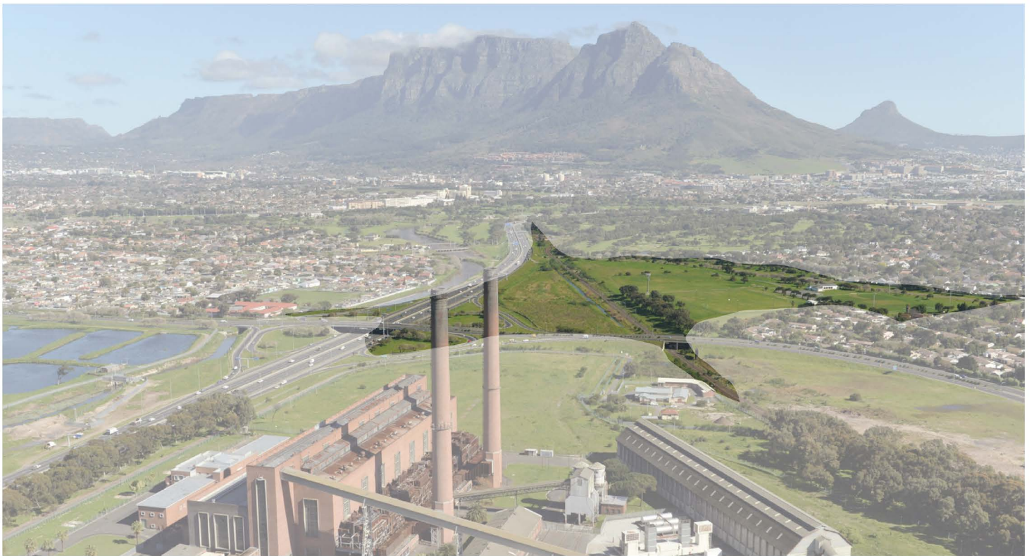
55: SHOWS AN AERIAL PHOTOGRAPH OF THE SITE EDITED TO HIGHLIGHT THE SITE IN CONTEXT WITH A VIEW OVER THE ATHLONE POWER STATION TOWARDS TABLE MOUNTAIN AND THE CBD.
