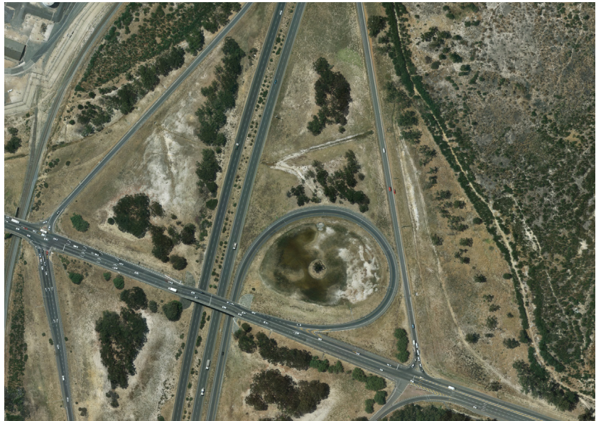
18: AERIAL VIEW OF PLATTEKLOOF ROAD OFF RAMP
