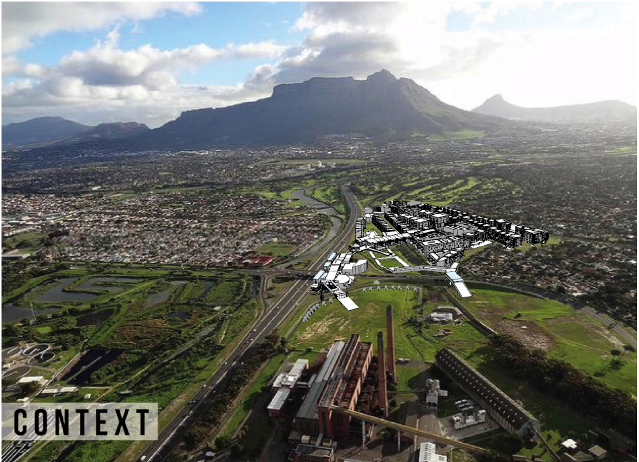
116: PHOTOGRAPH OVER SITE SHOWING PRELIMINARY SITE DESIGN IN PLACE
