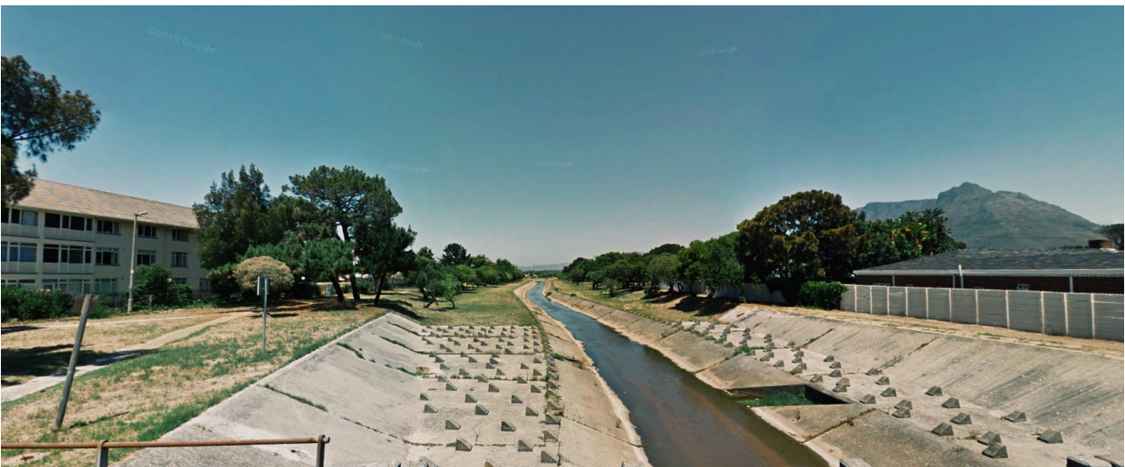
67: VIEW OF CANAL FROM NIGHTINGALE WAY BRIDGE
