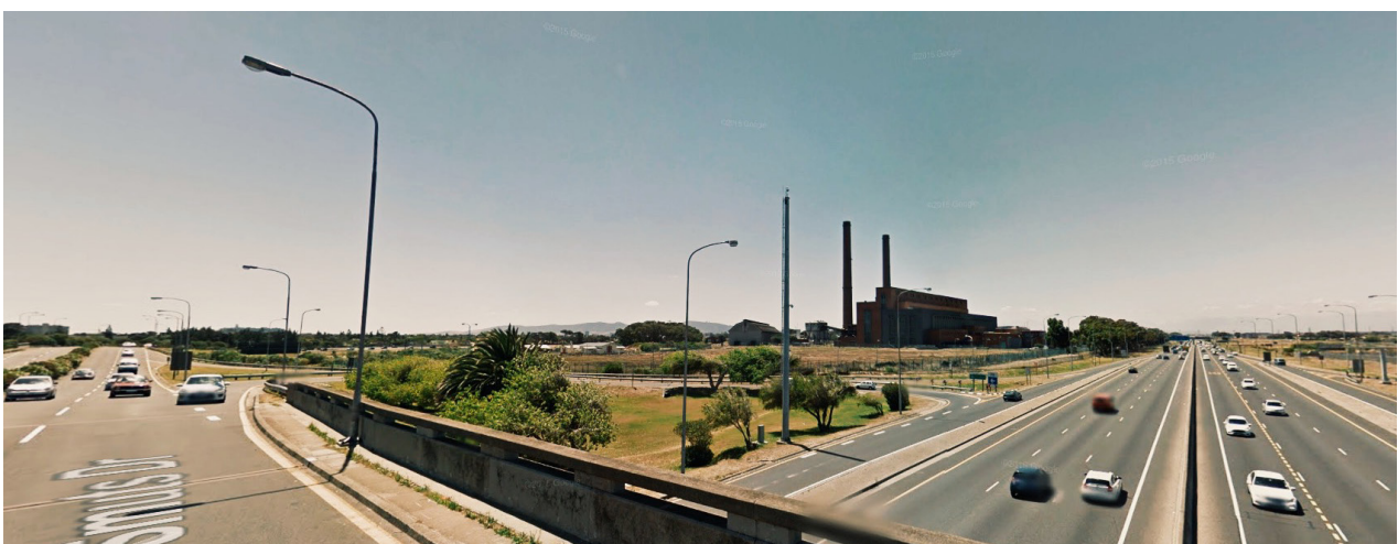
74: VIEW FROM JAN SMUTS OVER CLOVER LEAF TOWARD ATHLONE POWER STATION
