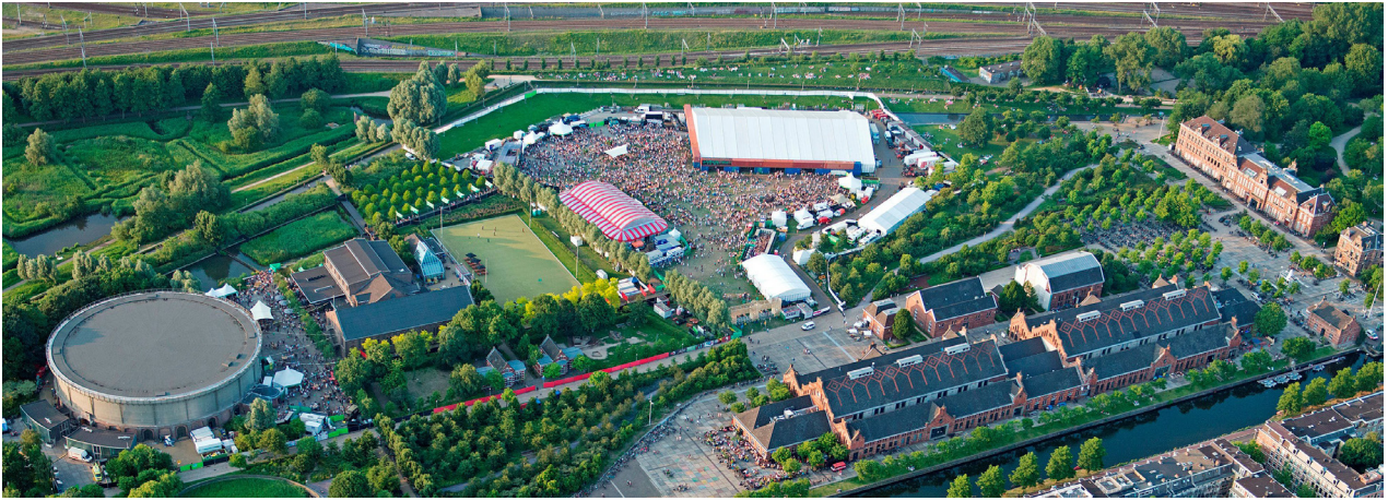
49: PRECEDENT IMAGE FOR THE REDEVELOPMENT OF THE ATHLONE POWER STATION SITE. WESTERGASFABRIEK, AMSTERDAM
