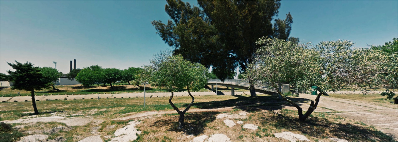
66: PEDESTRIAN BRIDGE FROM PINELANDS ONTO SITE
