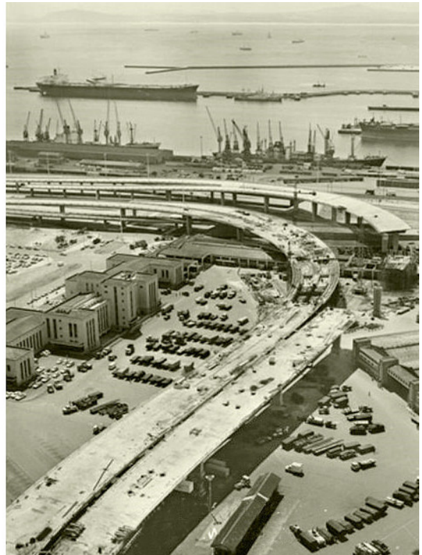
FORESHORE FLYOVERS TAKING SHAPE
