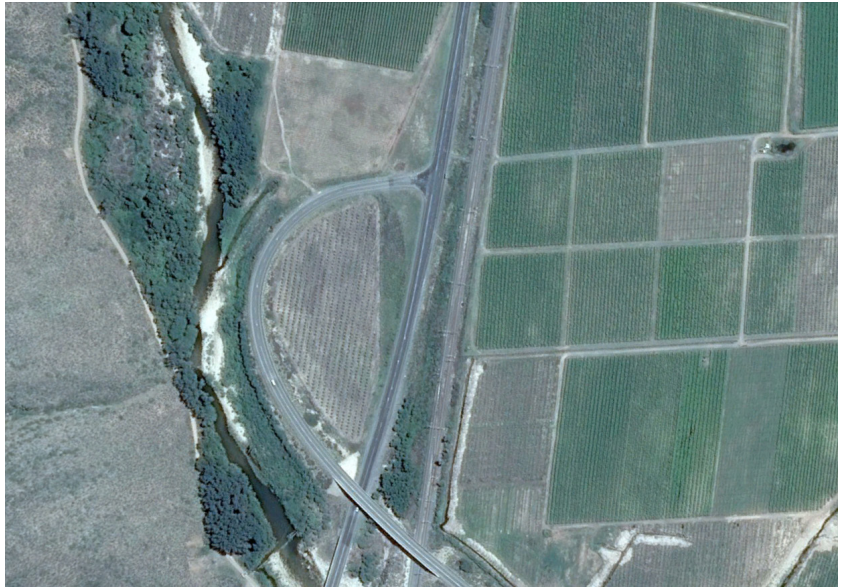
24: AERIAL VIEW OF OFF RAMP ALONG HEX RIVER
