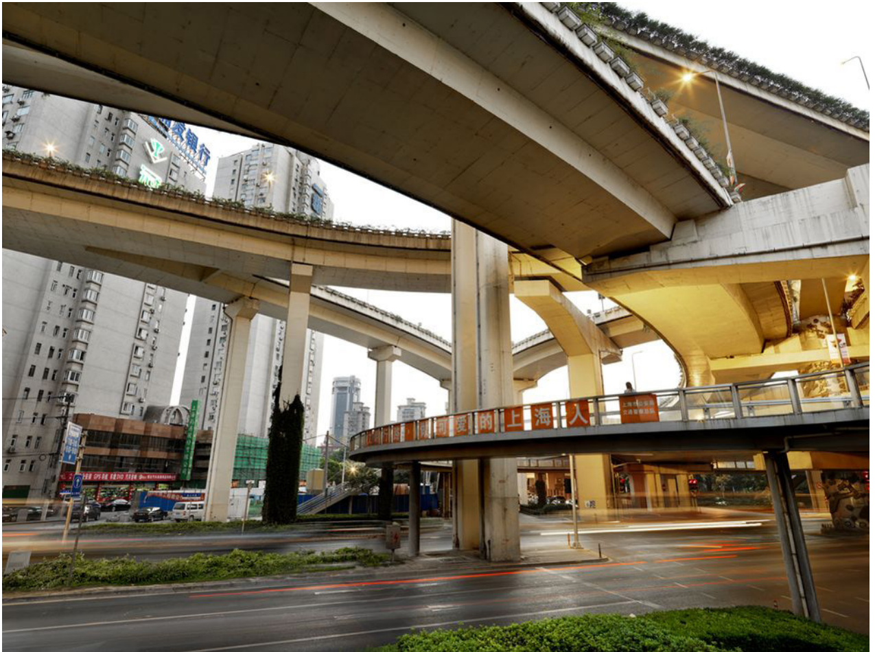
SHANGHAI ELEVATED HIGHWAY
