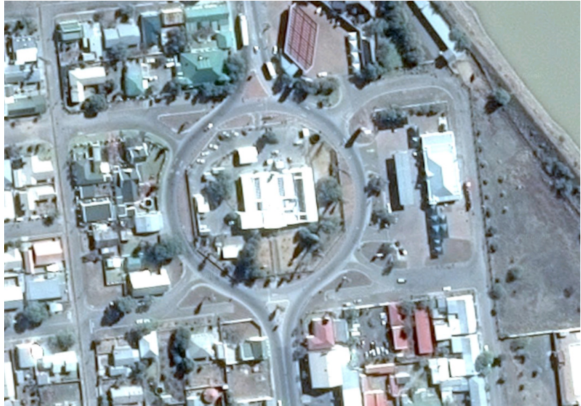
22: AERIAL VIEW OF BEAUFORT WEST N1 CIRCLE
