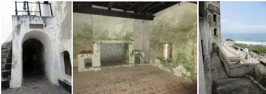
Figure 143. A neglected, ruin-like Elmina Castle. Source: author, 2016.
