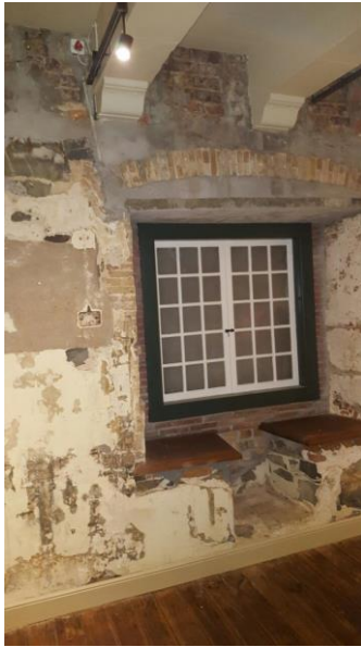
Figure 39. Restored room in the Castle of Good Hope showing the different layers of fabric (Source: author, 2016)
