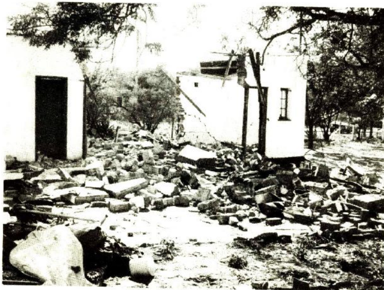
Figure 14: Building reduced to rubble , 1985. House number 5007, servants' quarters, Gaborone village; owner: Botswana Housing Corporation; tenant: Eugenia Kakale Kobole and Gladys Kelape Kesupile.
