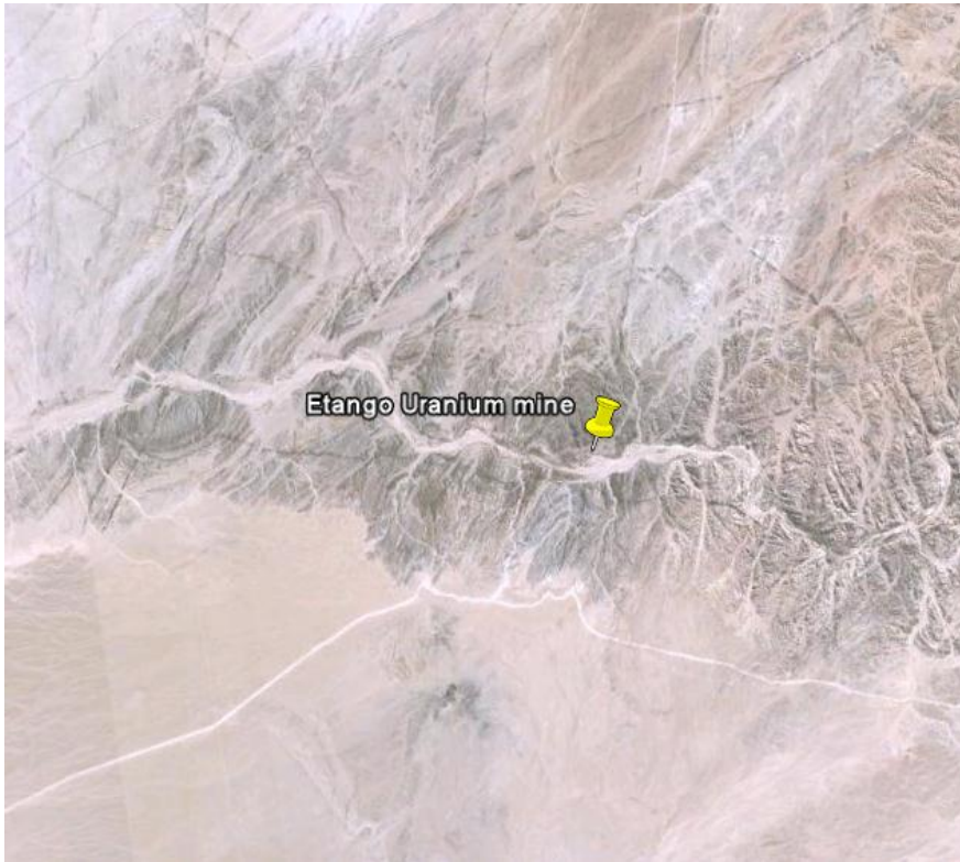
Figure 47: Aerial view of the Etango Uranium site (Generated using Google Earth, 2010)
