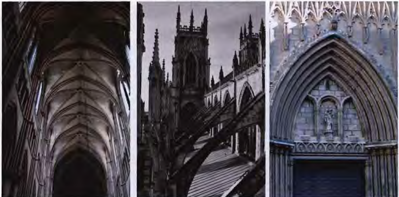
The three defining elements of the Gothic era of construction, the ribbed vault, flying buttress and pointed arch
