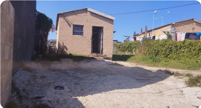
Authors own image PLANNED DUNOON PLOT The above image shows the original structure relating to a planned Dunoon which was a single story 6mx4m structure on a 15mx7.5m plot.
