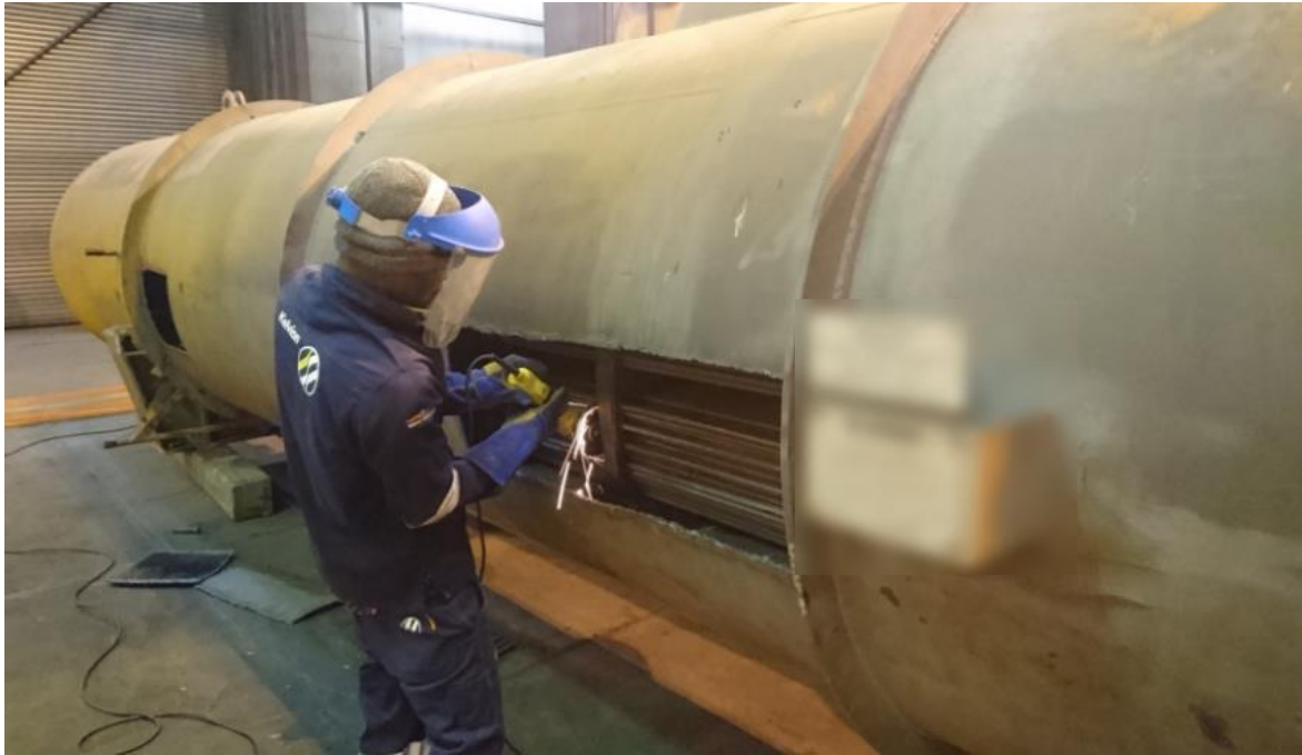
Figure 5-6: LP Heater Tube Sample Removal
