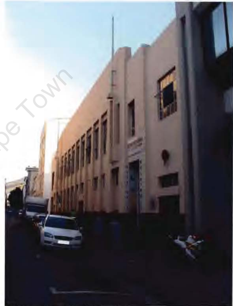
26 Commercial Street | Cape Town | 2007
