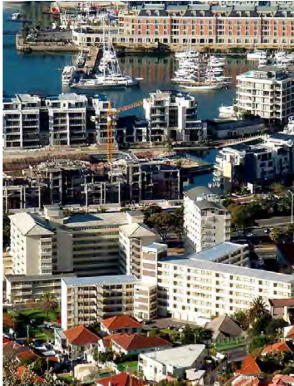
Figure 8.4: High-end apartment blocks in the Victoria and Alfred Waterfront Cape Town (Source; Fourie, 2010)
