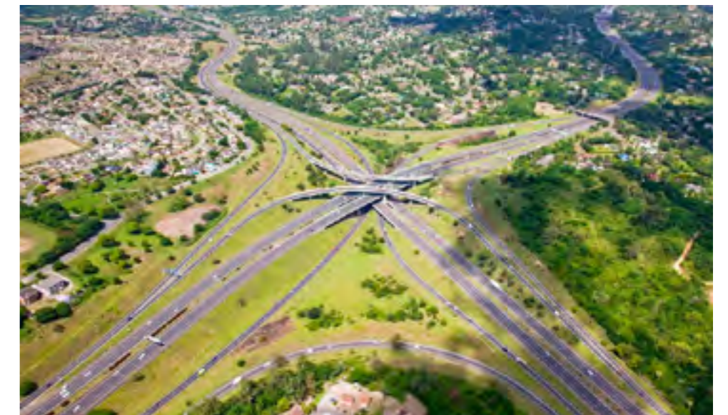
Figure 3.1 Spaghetti Junction in Durban: (Source; Pitcher, 2011)
