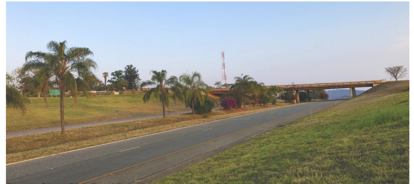
Fig. 41: Site 4 R71: Road Reserve
