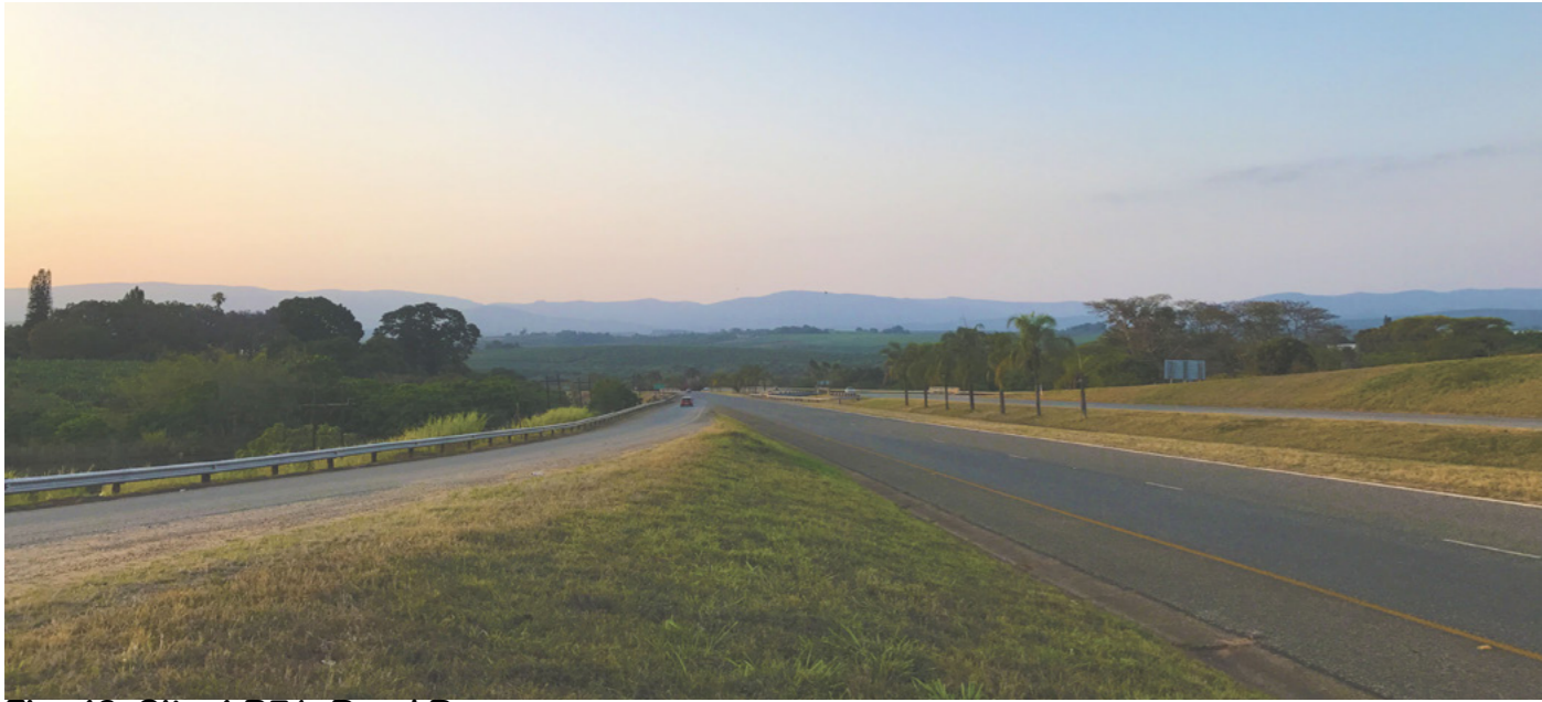
Fig. 42: Site 4 R71: Road Reserve
