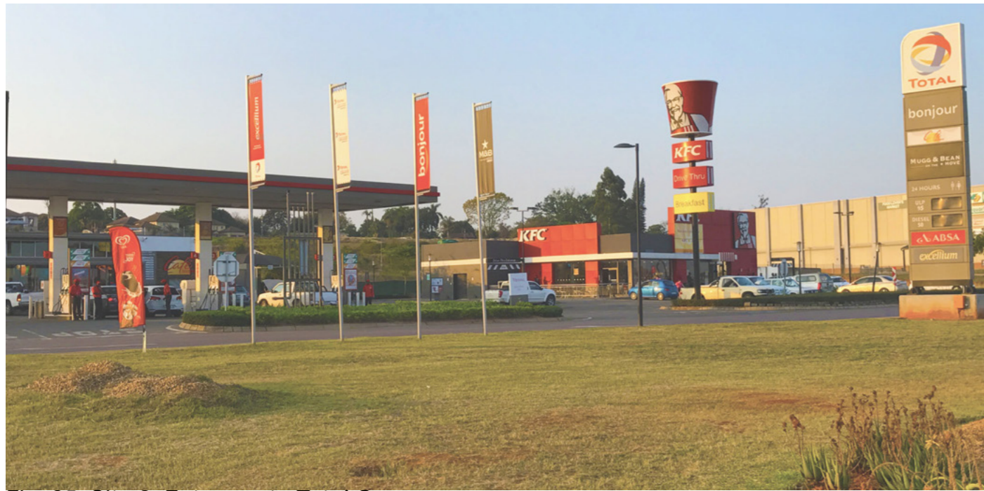
Fig. 25: Site 2: Entrance to Total Garage
