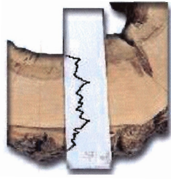
Figure 2.2: Resistograph Measurement showing decay [16]
