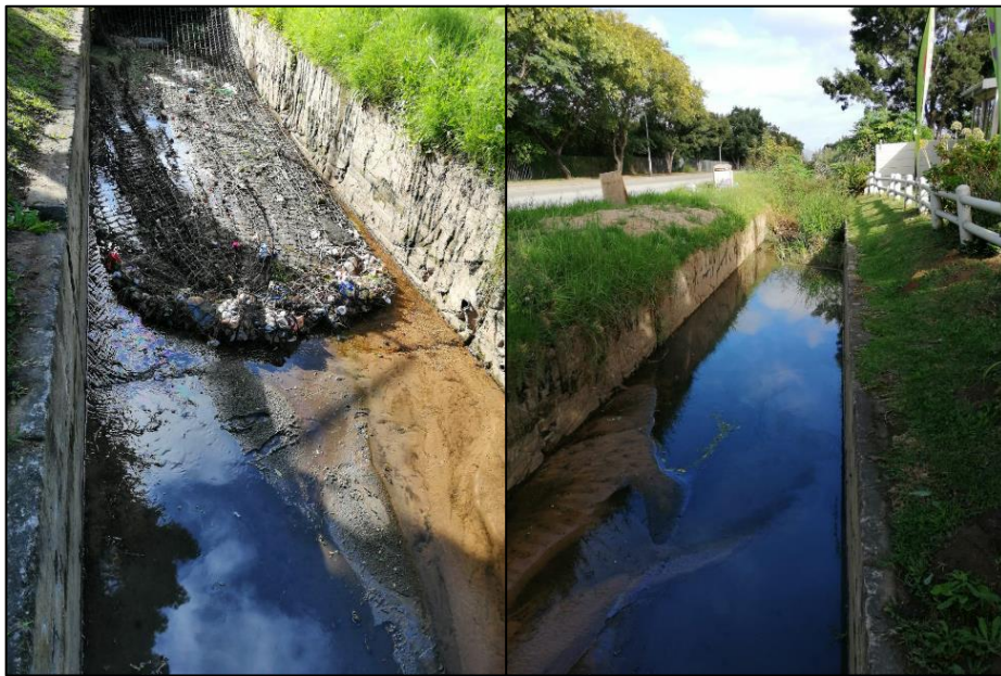
Figure 5.24: Photographs showing the litter net on Vigilance Drive (left), and the sampling site (right), located about five metres downstream of the net
