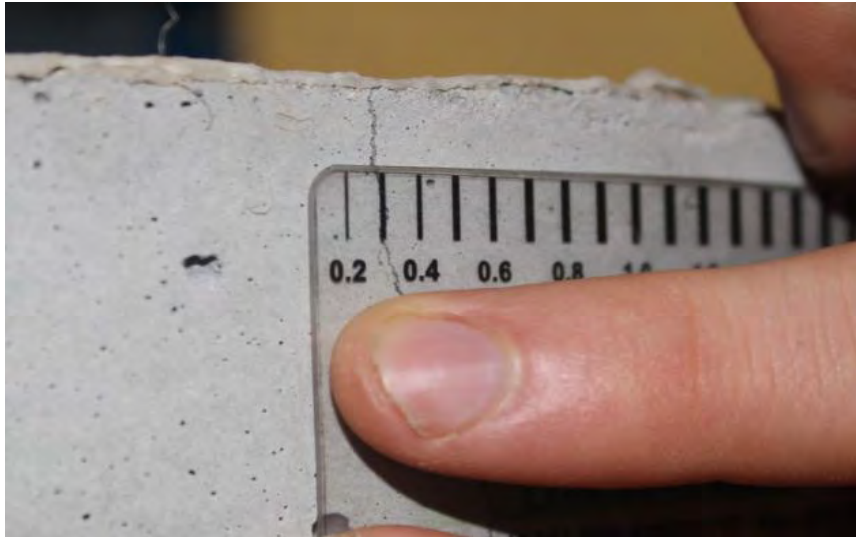
Figure 3.12: Using a crack card to measure crack width
