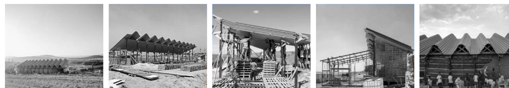
Figure 17: Images source: "Silindokuhle Preschool / Collectif saga" 25 Jul 2017. ArchDaily. Accessed 5 Apr 2022. < https://www.archdaily.com/875103/silindokuhle-preschool-collectif-saga > ISSN 0719-8884
