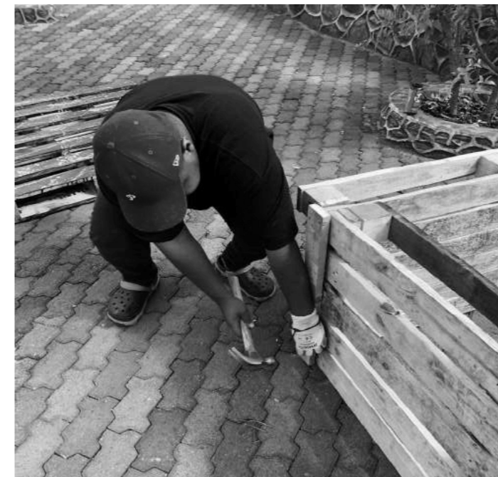
Images of the material prototype construction process taken by Author, 2022
