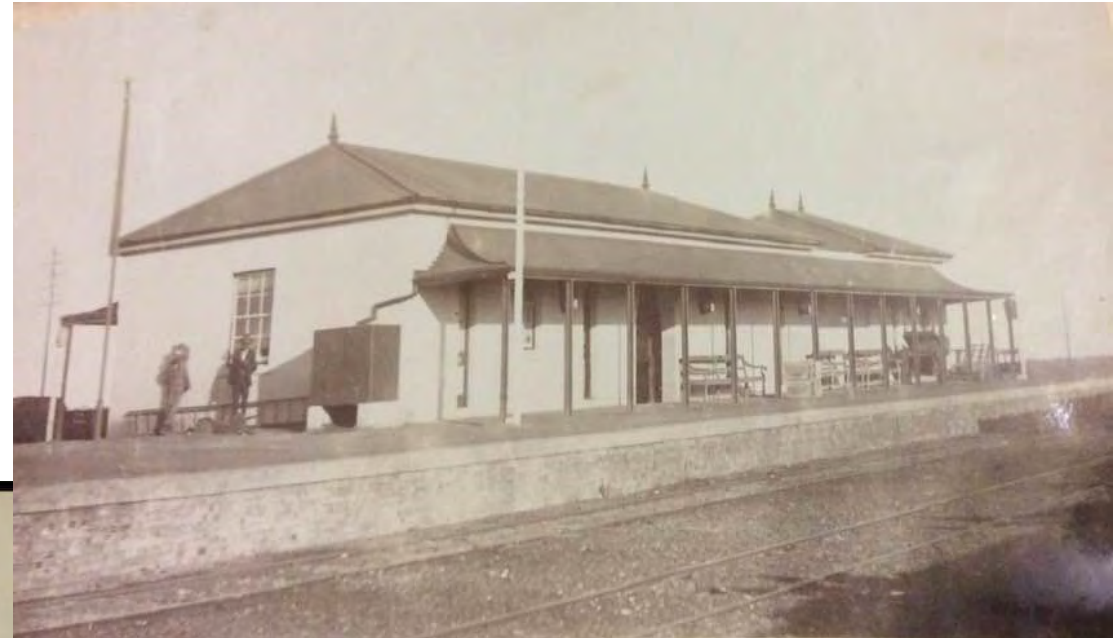
Figure 64: Swartkops Station in the early 1900s (Source: McClelland, n.d.)
