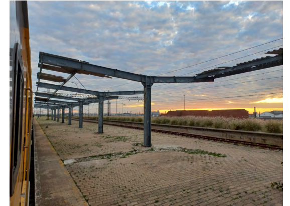
Figure 45: New Brighton Station (Source: Author, 2024)
