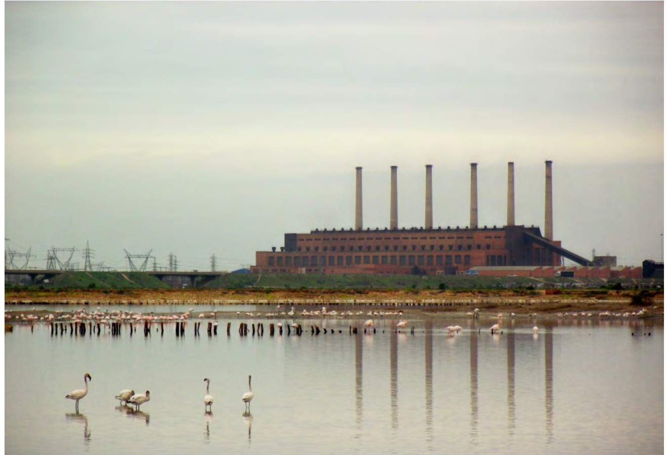
Figure 71: The Swartkops Power Station is a building of significance and heritage and has the potential to be re-imagined to become significant in its use to the community (Source: Fourie, 2013)
