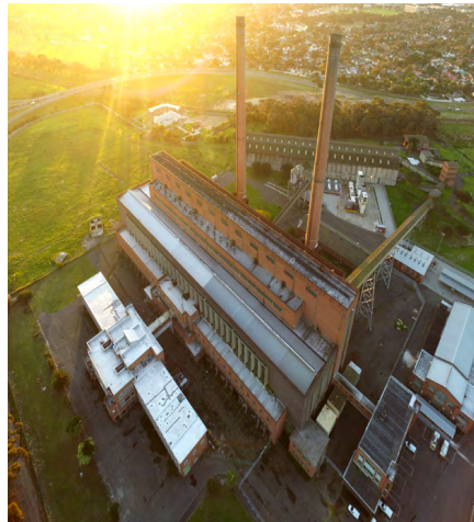
Figure 28: Athlone Power Station (Source: COCT, 2023)
