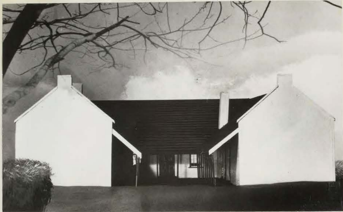
7. West facade of Drostdy, Bathurst, showing the interior Court and the veranda. (restored R.B. Lewcock, model, J.Y. Murray).
