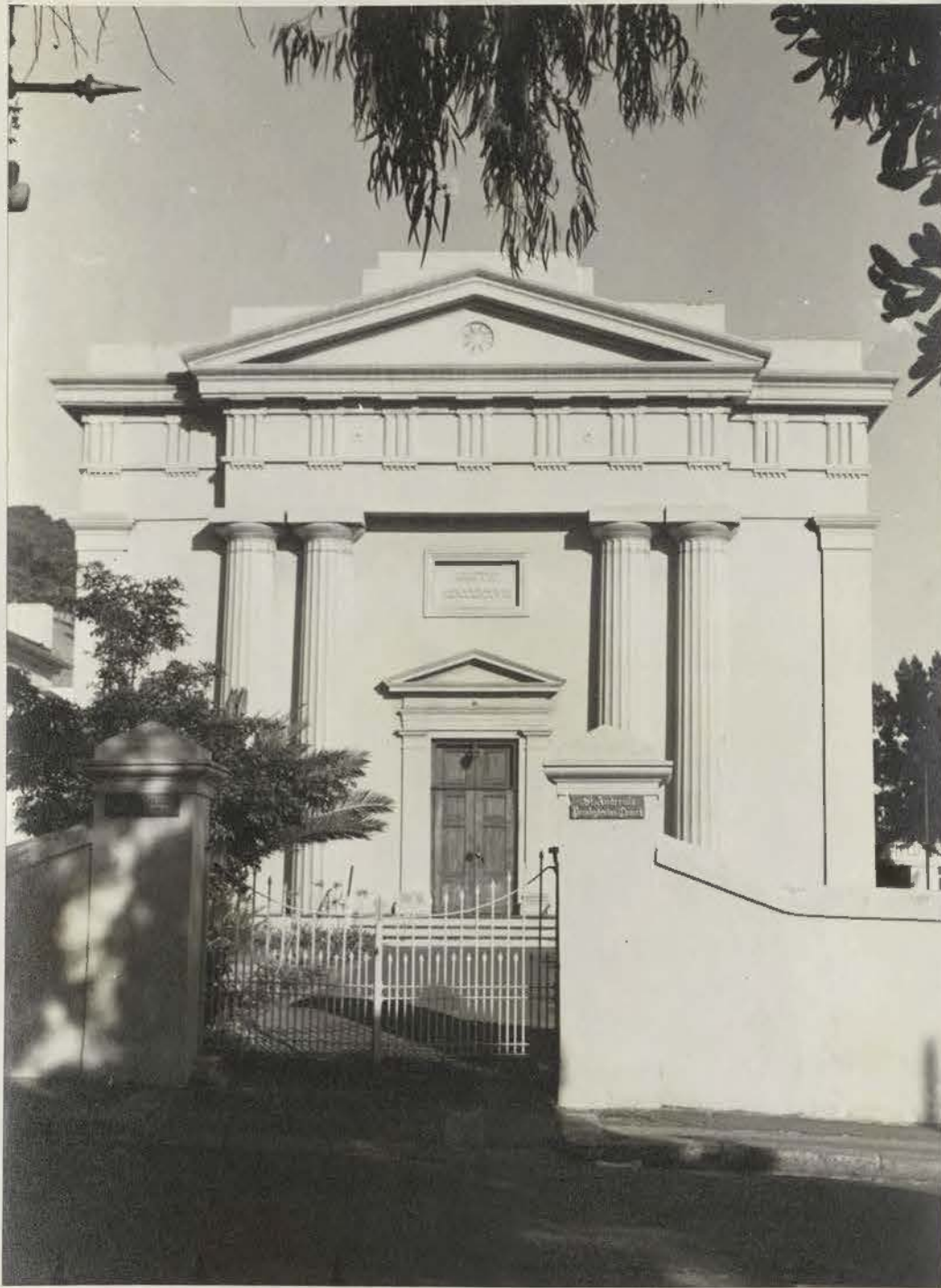
39. The facade of St. Andrew's Presbyterian Church, Cape Town, 1827-8.
