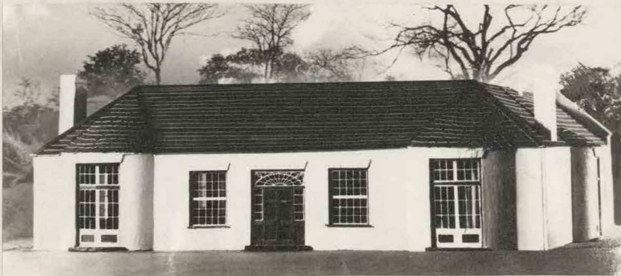
6.B. (Below). Entrance (East) facade of the Drostdy, Bathurst (restored R.B. Lewcock, model, J.Y.Murray).
