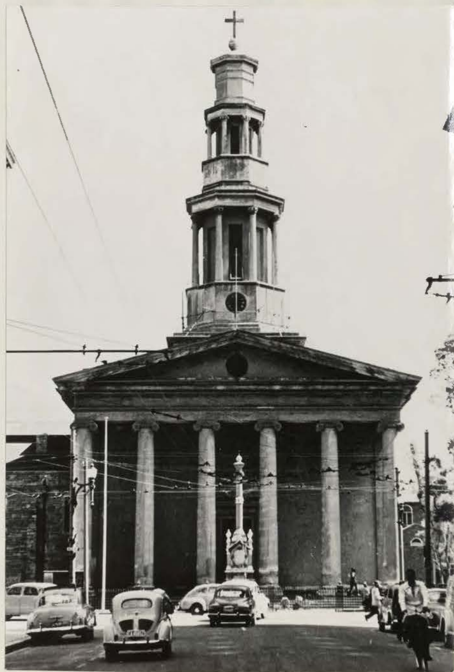
38. The facade of St. George's immediately before demolition.
