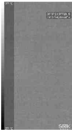
(a) IR image of the inner wall.
