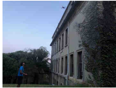
(b) Northern Side wall.
