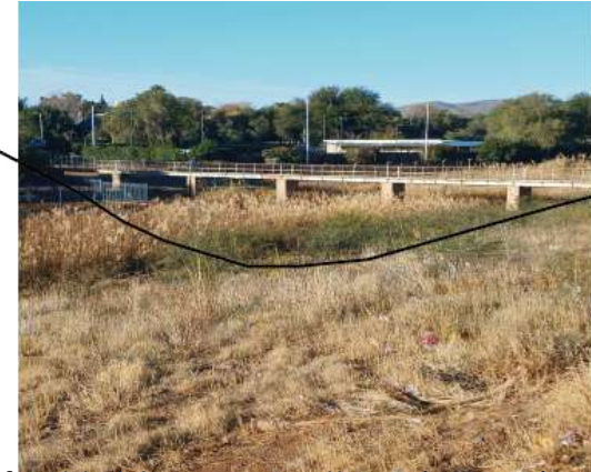
Oldest foot bridge across the Prieska River.
