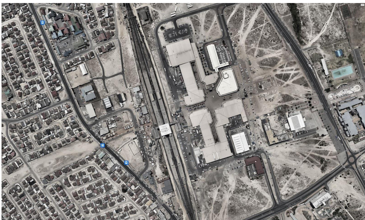
Figure 11: Satellite image of Khayelitsha Station and surrounds (Including Khayelitsha Mall) (Google Earth, 2023)
