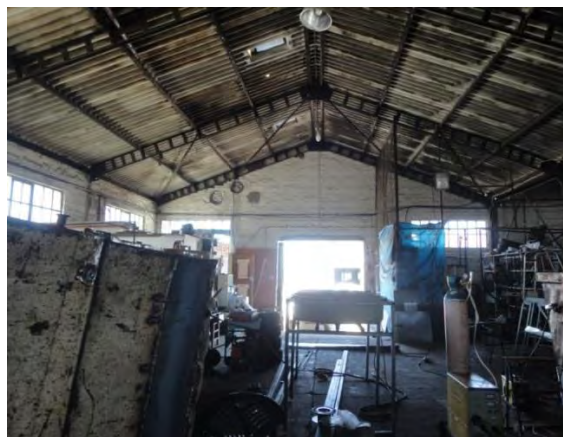
Figure 154: The steel frame is visible on the inside (Author, 2013)
