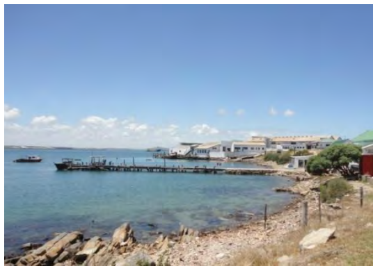
Figure 229: Timber pier in Saldanha Bay (Author, 2013)
