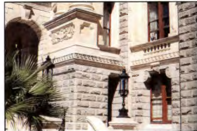
Figure 19: Beige limestone and light grey granite, from the Glencoe Quarry - Cape Town City Hall
