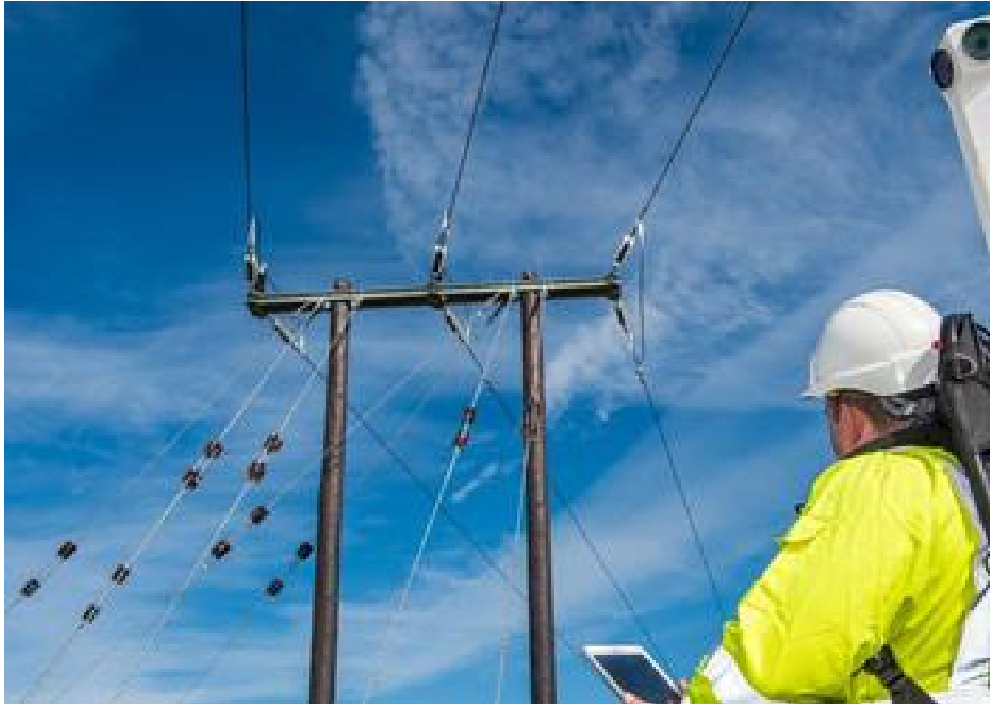
FIGURE 2.2: Foot patrols as means of inspection.
