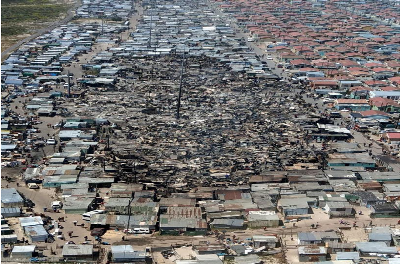
Figure III: A picture showing an aftermath of a fire incident in Silvertown (Source: Smit, 2018).
