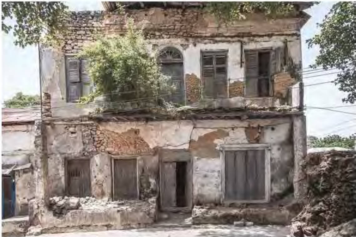
Double storey stone house ruin, open carved Zanzibari door, timber shutters, coral and limestone building construction, tree growing in upper level Ocean Road, Bagamoyo, 11 June 2015
