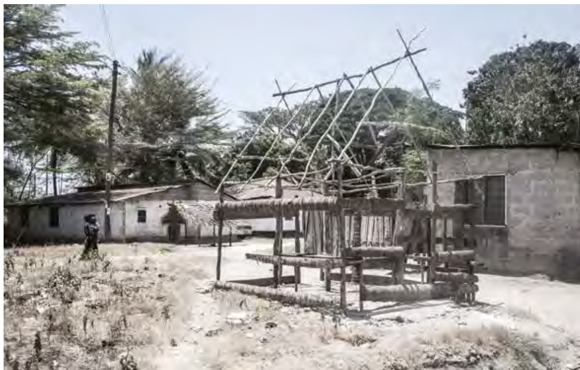
Path, timber structure, prospective retail unit Bagamoyo, 26 September 2015
