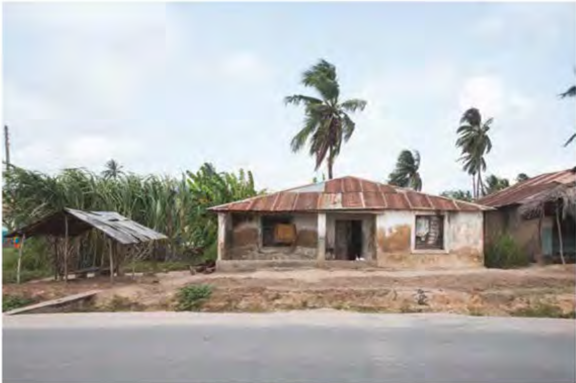
Typical Swahili residential typology, central timber door with view of rear yard, entrance porch, raised front veranda, modular tin sheet roof double hipped pitch, 2 symmetrical windows and frames; Maputo style Bagamoyo, 16 June 2015
