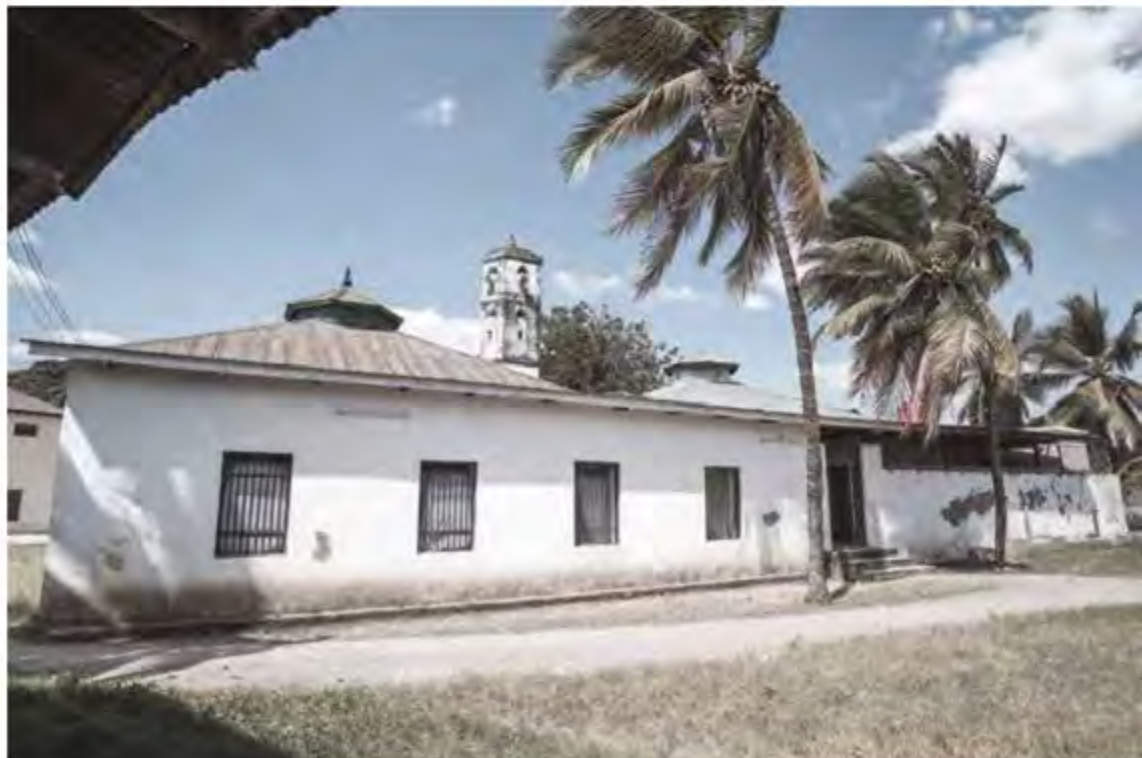
The Ibadi Gogoni Mosque , building extensions, palm trees, Bagamoyo 13 June 2015
