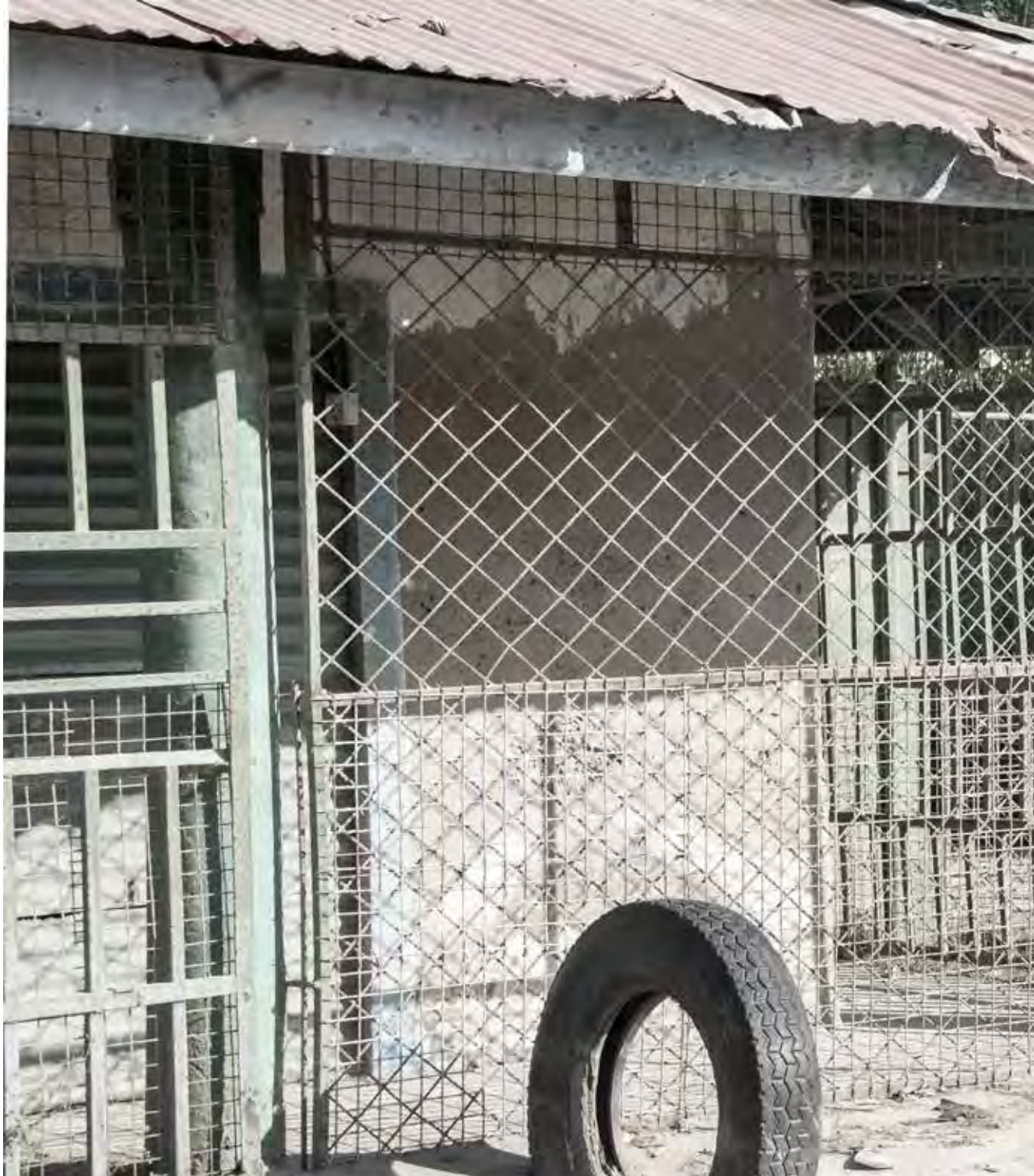
Security screens, mesh, secondhand rubber tyres, sheltered outdoor area, defining territory Bagamoyo, 13 June 2015
