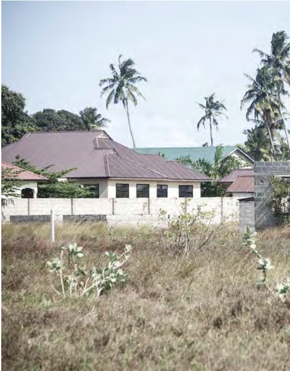
Palm and mango trees close to Mrisho Kikwete Drive. Residential dwellings under construction. Cleared tropical bush to foreground Ukuni, Bagamoyo, 27 September 2015
