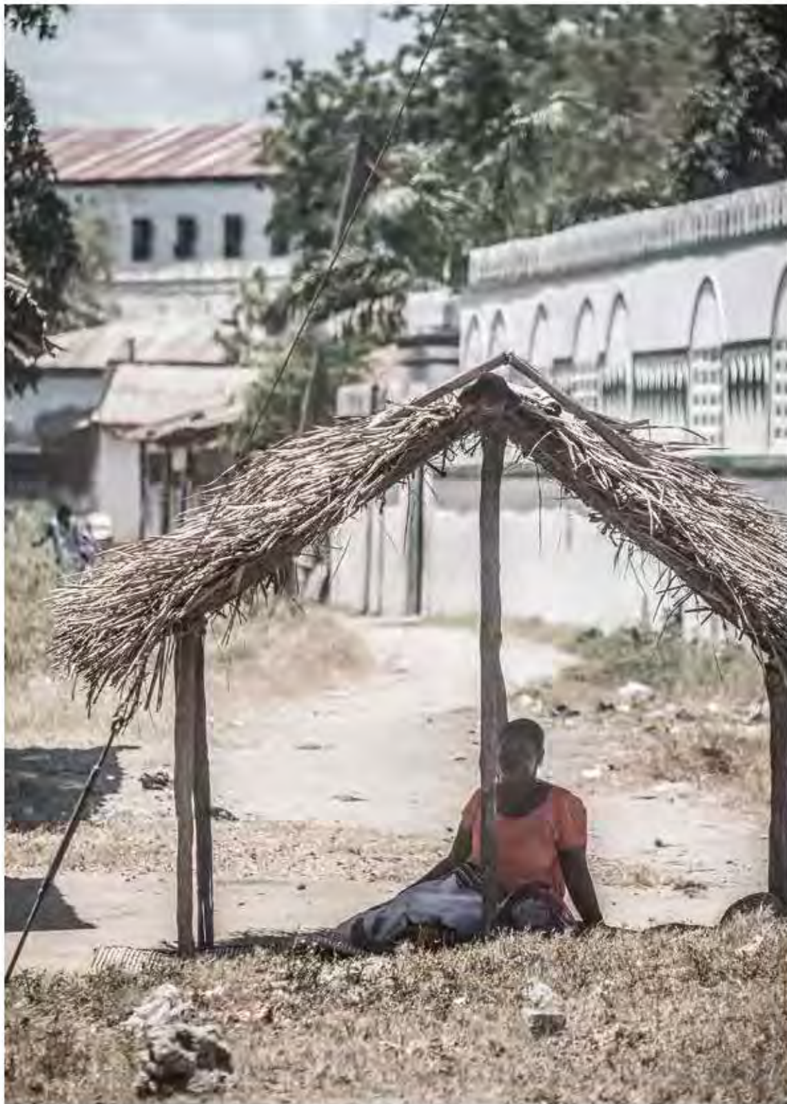
Independent baraza of palm leaf with timber pole construction, providing shelter, along public path with entrance to Shia Ithna Asheri Mosque Bagamoyo, 27 September 2015
