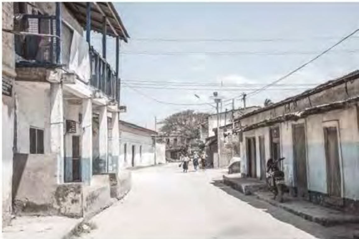
Residential buildings, Old Market road, Bagamoyo 2015 22 September 2015
