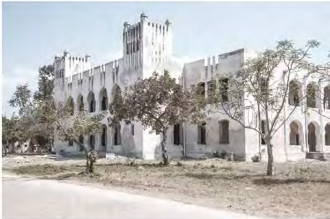
Unoccupied undergoing refurbishment, Ocean road, Bagamoyo 22 September 2015
