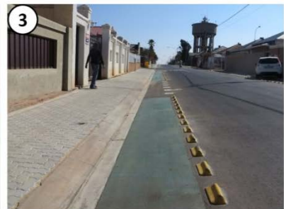
Quiet residential street with rumble strips in Brixton (Source: JUCA)
