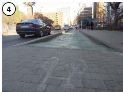
Kerbed separation between cyclists, vehicles, and pedestrians (Source: JUCA)
