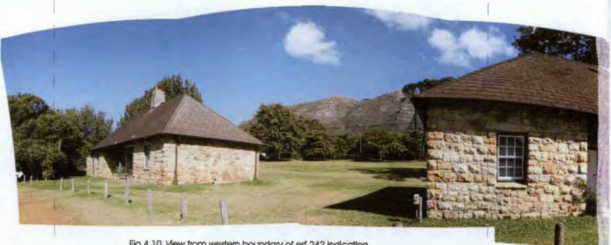
Fig 4.10. View from western boundary of erf 242 indicating stone cottages (by author ,2010)
