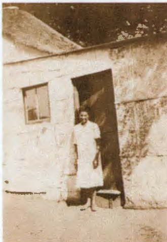
Fig 2.9. Typical extension to the main house (D6 museum)
