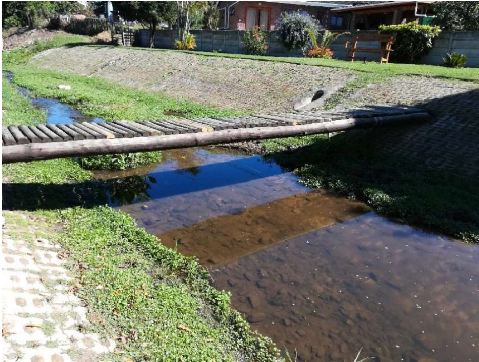
Figure 3-19: Bongani River water level monitoring point 4b
