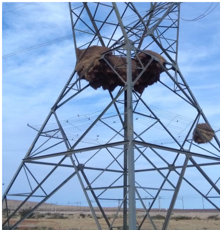
Figure 10: Sociable weaver nests on a transmission line tower, Northern Cape, South Africa. Photo credit Corey Jeal
