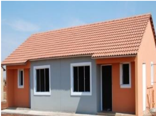
Left: Breaking New Ground house. Source: Joburg.co.za
