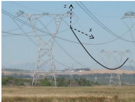
Figure 1.4: Reference frame with x axis along the line and z axis up [1].
